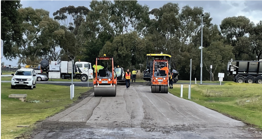
VU researchers are working on recycled material road onsite.
