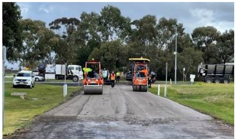
VU researchers are working on recycled material road onsite.
